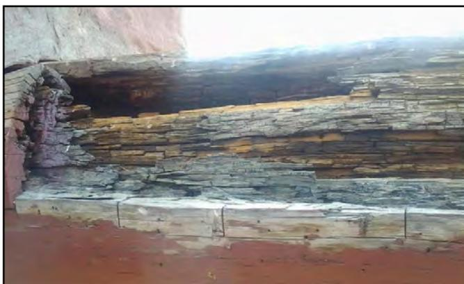
**Photo (left): Rotting support log on the Council Chamber.**
