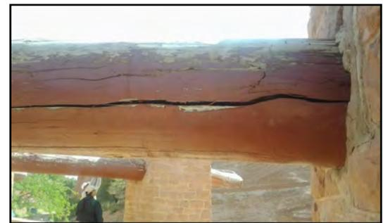
**Photo (above): Deteriorating support log on the Council Chamber.**
