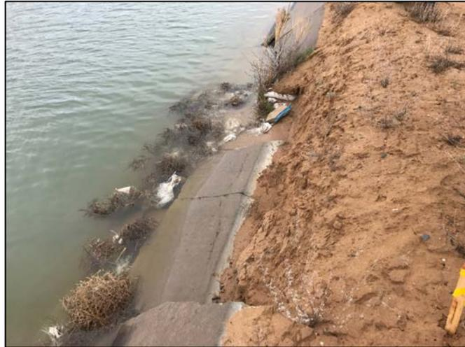
**PHOTO: A portion of the deteriorated water canal at the Navajo Indian Irrigation Project.**
