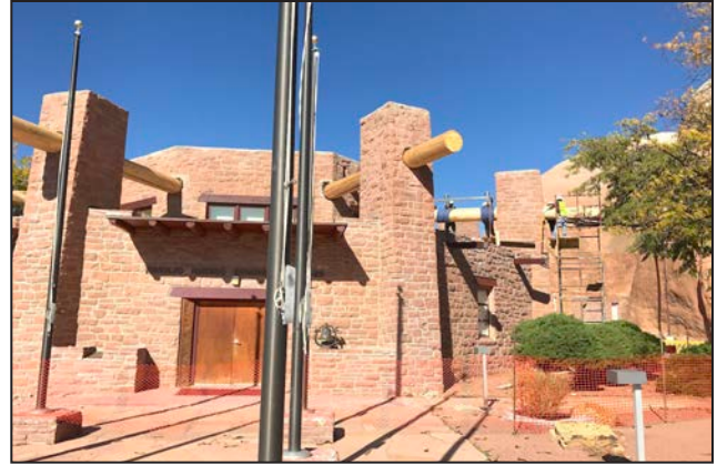
PHOTO: Newly installed permanent log beams on the Council Chamber.
