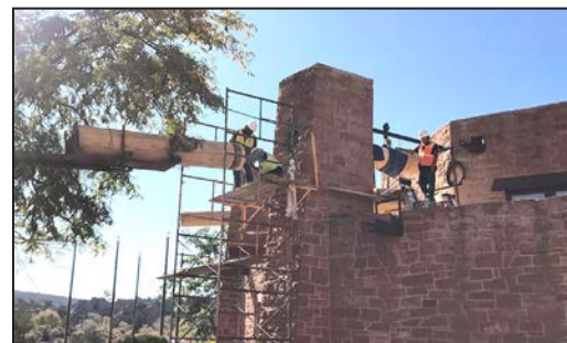
PHOTO: Workers installing the permanent log beams onto the Council Chamber
