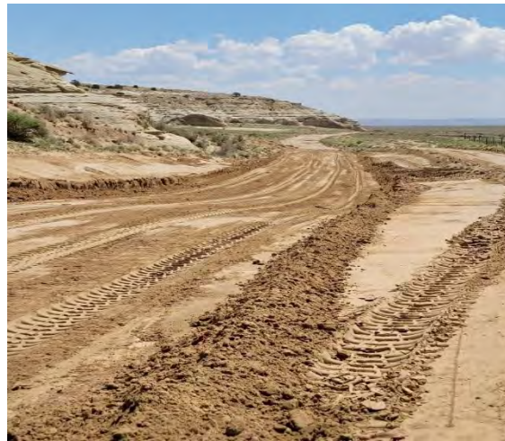
AFTER – Route N25: Erosion areas repaired.
