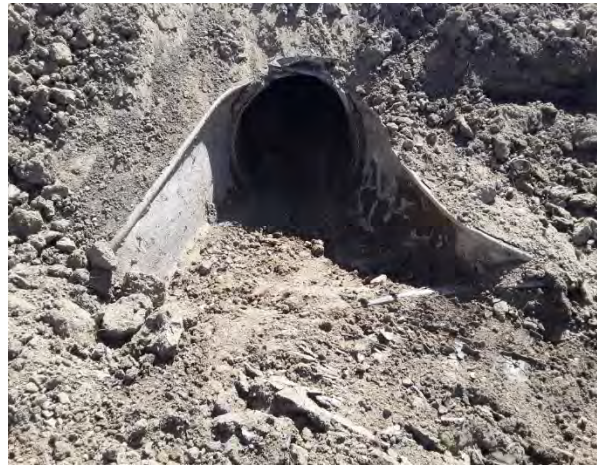
AFTER – Route N59: Exposed and Cleaned Pipe
