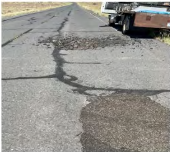
BEFORE – New Lands Road: Pavement Surface Damaged AFTER – Roadway surface repaired using UPM.
