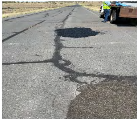
BEFORE – New Lands Road: Pavement Surface Damaged AFTER – Roadway surface repaired using UPM.
