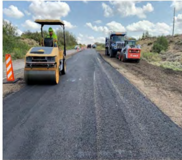
DURING – N3003: Compacting and finishing the new
