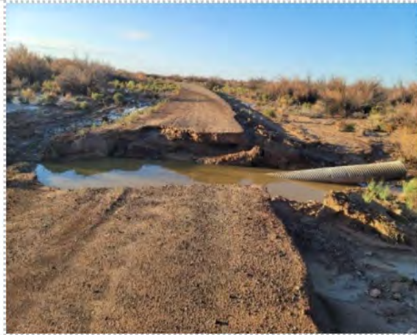
Monsoon 2021 – Western Navajo Agency Earth Road Repair: Install new pipe culverts.
