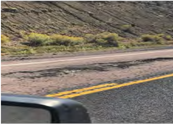
BEFORE – Route N12: Failed section of roadway.
