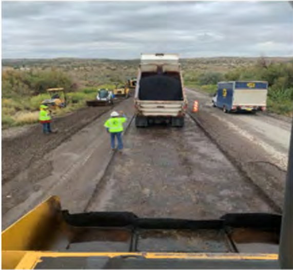
DURING – N3003: Mill and Fill Operation. Milled area. HACP.
