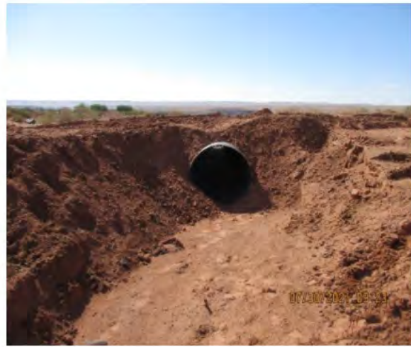
Monsoon 2021 – Western Navajo Agency Earth Road Repair: Install new pipe culverts.
