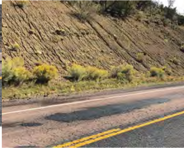
AFTER – Route N12: Pothole patching using UPM.
