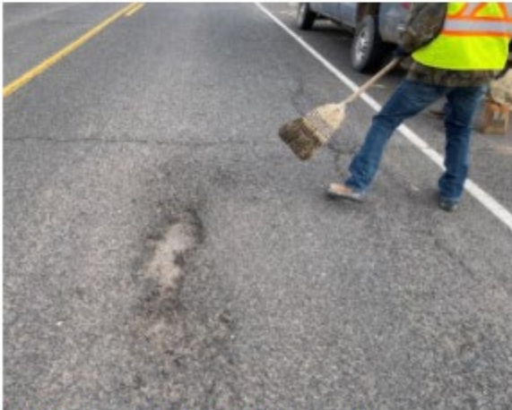
BEFORE: Route N64 - Patching preparation.
