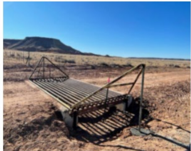
AFTER: Cattleguard installation/repair complete.
