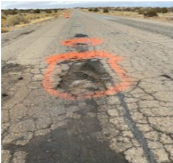
BEFORE: N3003: Damaged Roadway (Potholes).
