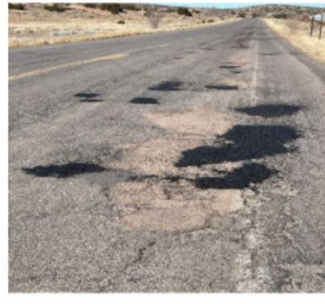
AFTER: Route N112 – Pothole Patching.
