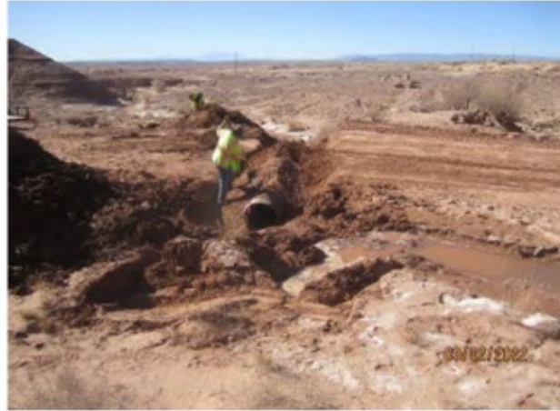
DURING: New culvert pipe being installed by crew.
