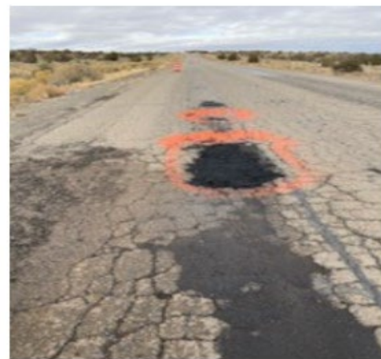
AFTER: Pothole Patching.
