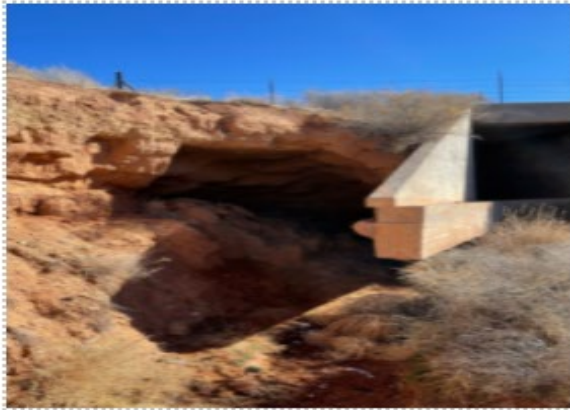
BEFORE: N6 - Erosion Repair under CBC Wingwall
