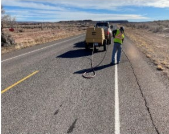
BEFORE: Route N27 - Cleaning crack using Air Comp.
