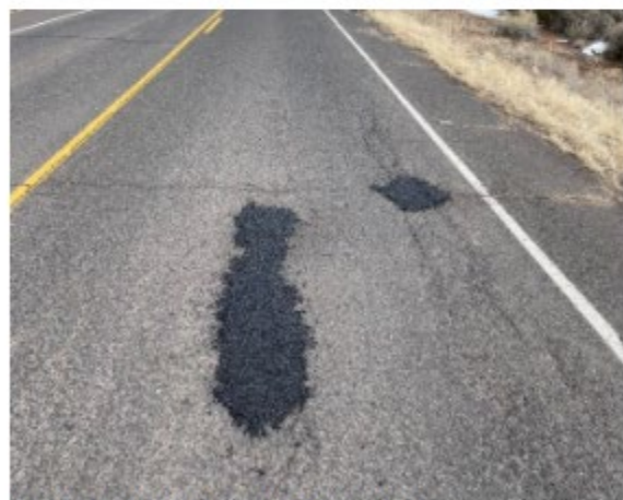
AFTER: Route N64 - Pothole patching
