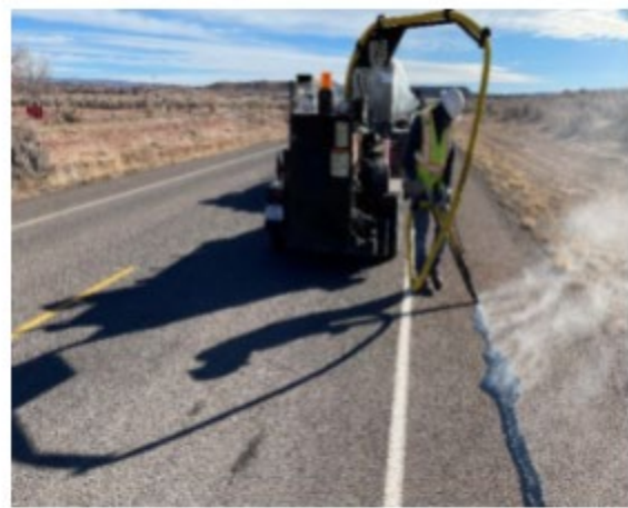
AFTER: Route N27 - Crack Sealing
