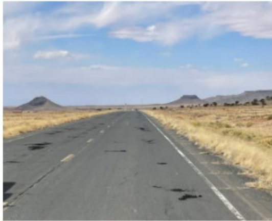
AFTER: Route N15 – Pothole Patching.
