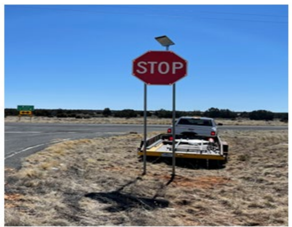
AFTER: NEW LED STOP sign installed.
