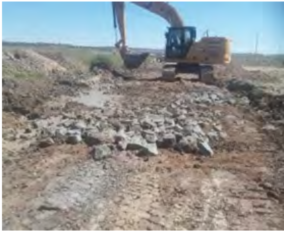
DURING: N8066- Washout repair.
