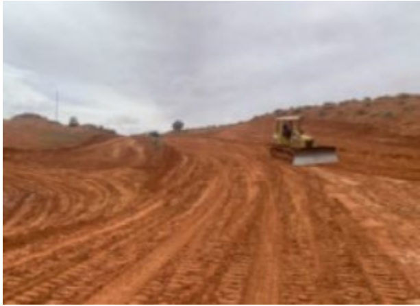
Earth road repair work on BIA Route N5037.
