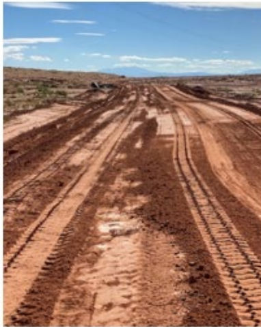
Storm runoff overtopped and eroded the roadway; backfilled roadway embankment on BIA Route N6731.
