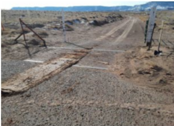
Cattle guard full of silt and debris; Cattle guard cleaned out on N59
