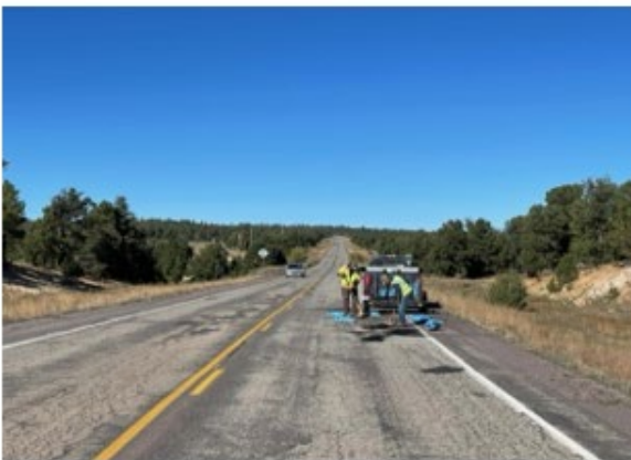
Pothole patching on N7
