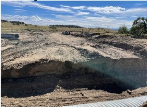
Storm runoff overtopped and eroded roadway on N30
