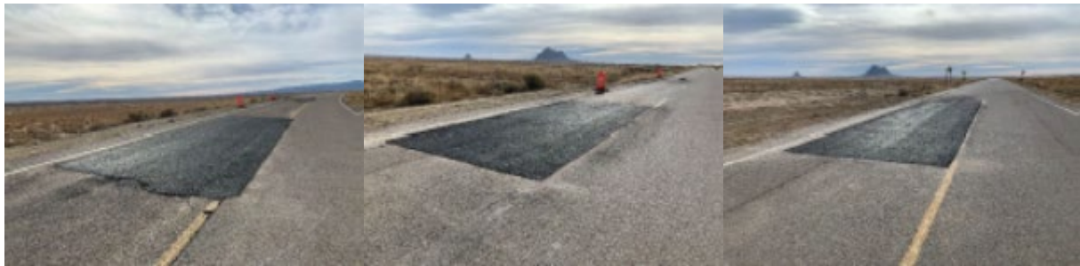
The Contractor that used this route as a haul route repaired the damaged sections of BIA Route N5000
