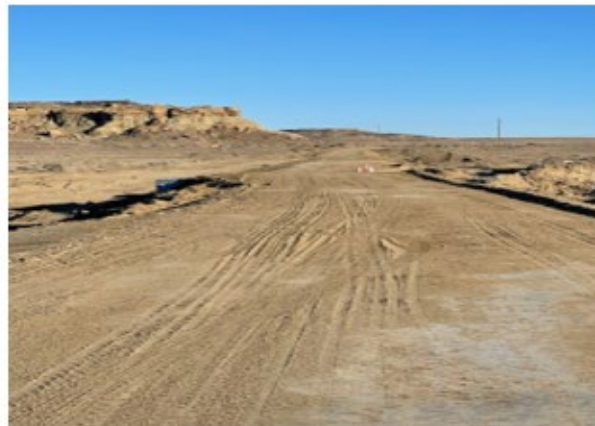
Backfilled roadway embankment on N9653
