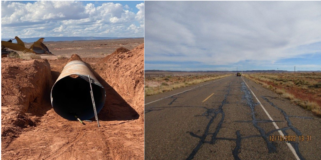
Culvert pipe replacement on BIA Route N23.
