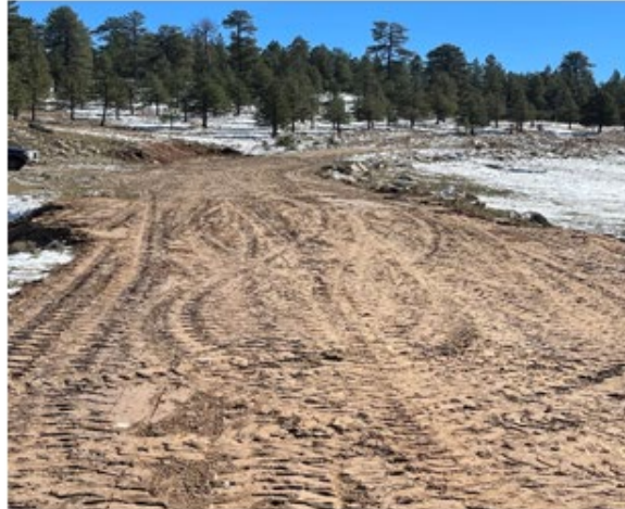
Backfilled erosion around pipes on N30
