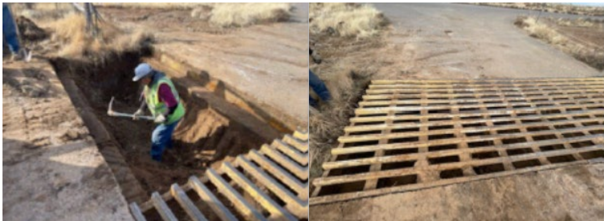
Cattle guard clean out work completed on BIA Route N3002
