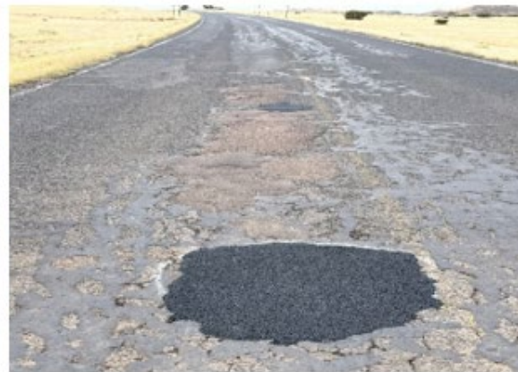
Pothole patching on N7
