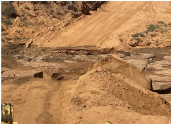
Existing earth road washed out on BIA Route N6310
