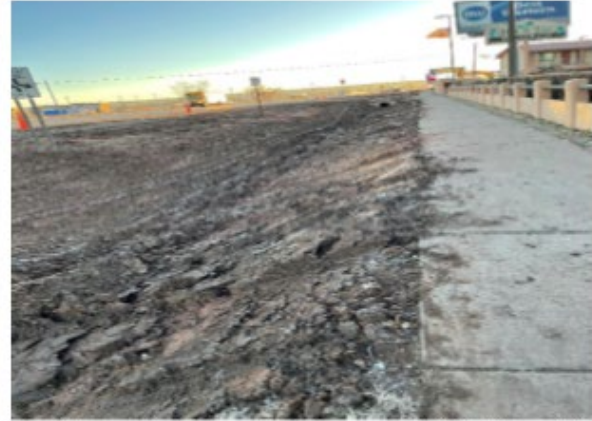
After: Removal of silt and debris; re-establish ditch on N7
