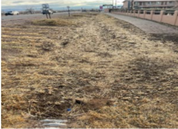
Before: Ditch full of silt and debris on BIA Route N7
