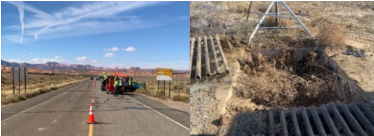
Pavement crack cleaning and sealing operation on Route N13 - Cattle guard clean out on BIA Route 36
