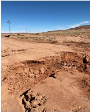
Storm runoff overtopped and eroded the roadway; backfilled roadway embankment on BIA Route N6731.
