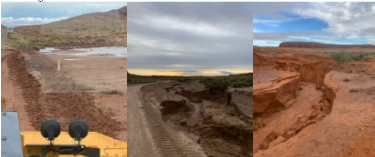
Earth road wash out on N12/US491. Severe erosion along BIA route N351. Severe erosion and road washout on N5043.
