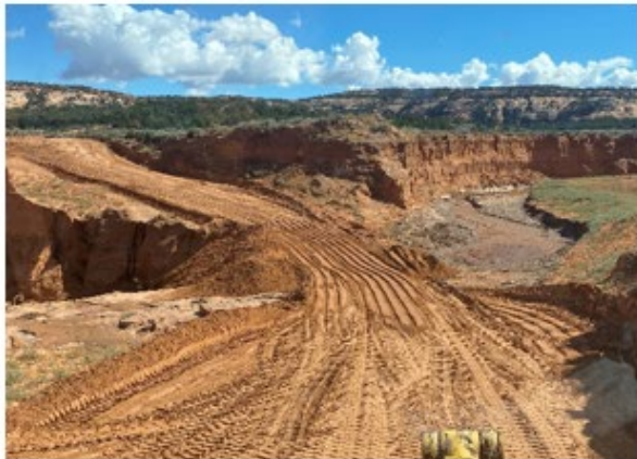
Backfilled road embankment to provide access on N6310
