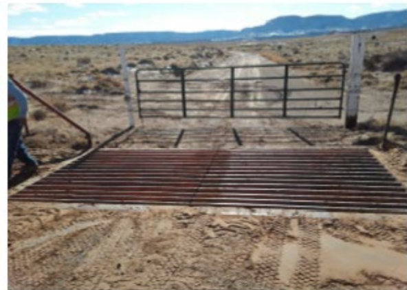
Cattle guard full of silt and debris; Cattle guard cleaned out on N59
