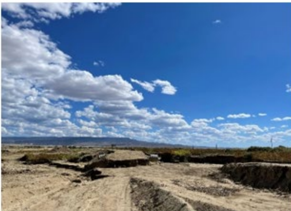
Storm runoff overtopped and eroded roadway on N9653
