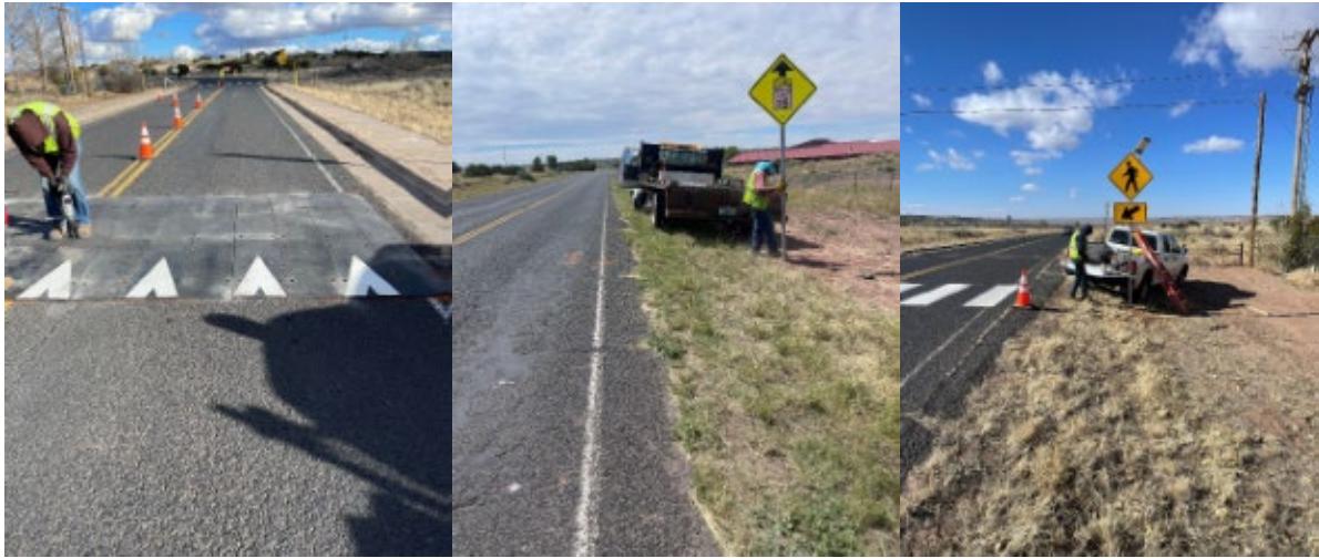
Speed hump installation, school speed limit and pedestrian crossing warning signs installed on BIA Route N2011
