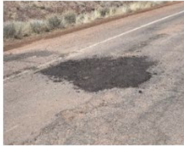
Pothole Patching on N112
