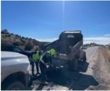
Pothole Patching on N112
