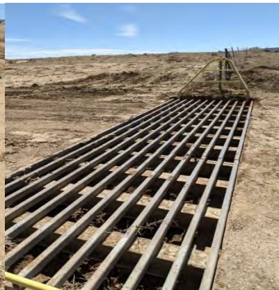
N9 – Cattleguard cleanout during and after.
