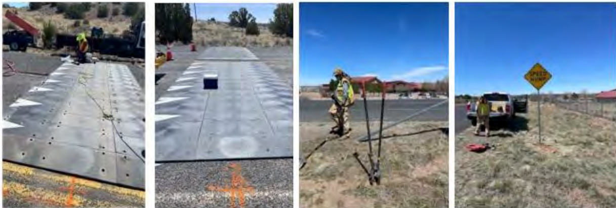
N2011 – Speed hump & “Speed Hump” sign installation in school zone before, during and after.
