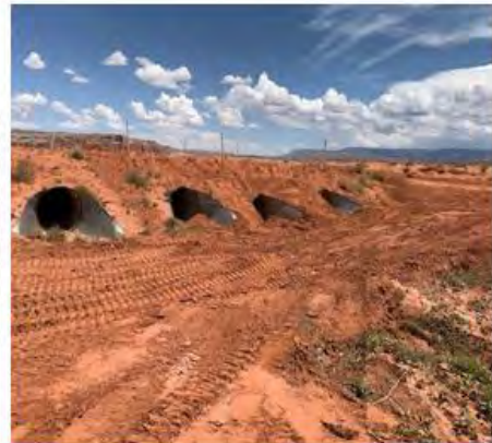
N5054 Repair Work. N5054 Repair work complete. N5054 Culvert pipes were reinstalled.
