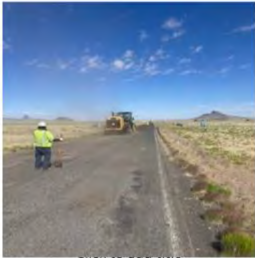
N602 – Pavement preservation during milling, base repair, and paving.
