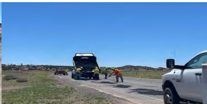
N112 – Pothole patching during and after.
