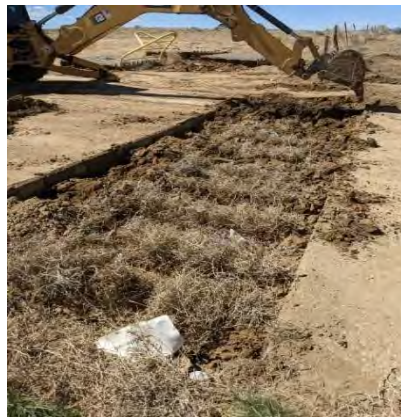
N9 – Cattleguard cleanout during and after.
