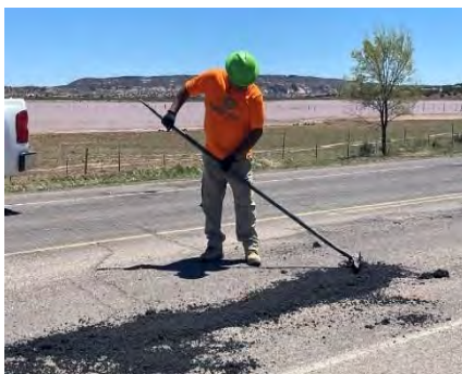
N112 – Pothole patching during and after.
