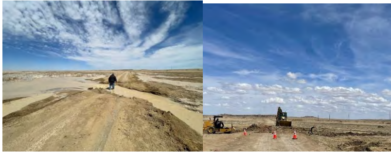
N9653 – Culvert pipe washout repair before and after.
