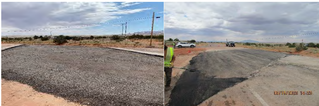
N6331 – Place new Aggregate Base
