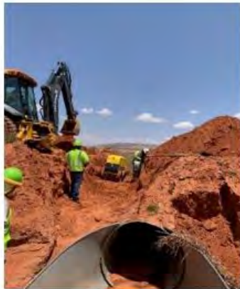
N5054 Repair Work. N5054 Repair work complete. N5054 Culvert pipes were reinstalled.
