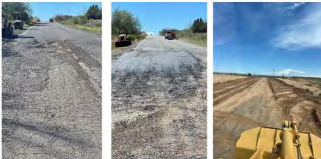
N3003 – Pavement surface repair before and after. N4073-Shoulder maintenance & sand removal.
