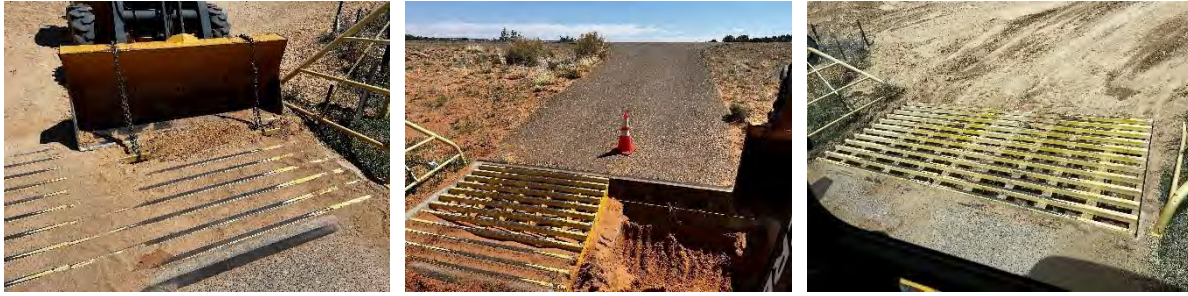
N21-Cattleguard cleanout before N21-Cattleguard cleanout during N21-Cattleguard cleanout after.
