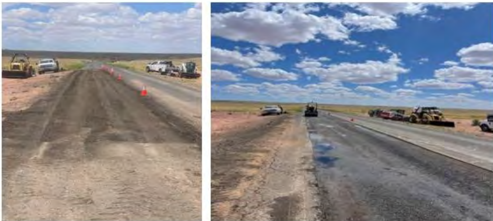
N60 – Pavement preservation during milling, base repair, and paving.
