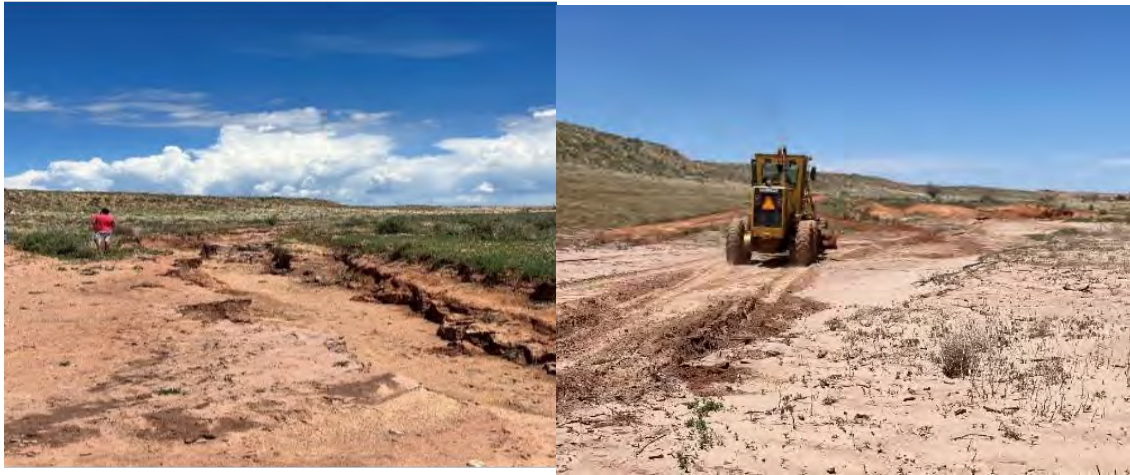
N157 – Washout repair before and after.
