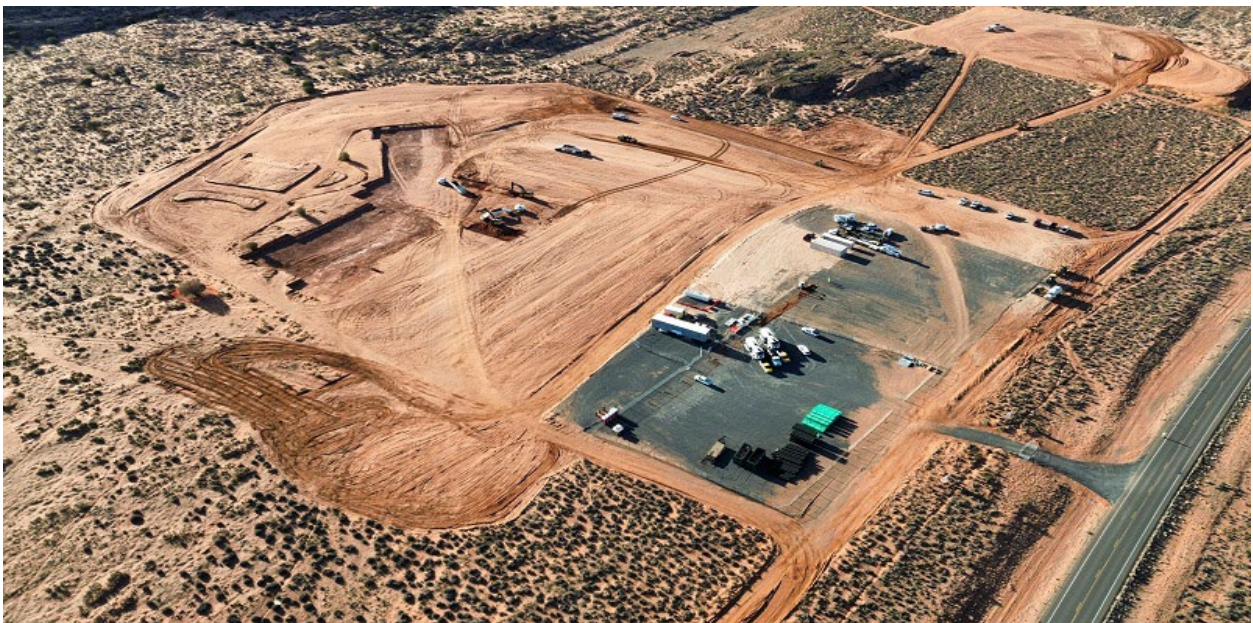
Drone photo of the future BGHC site
