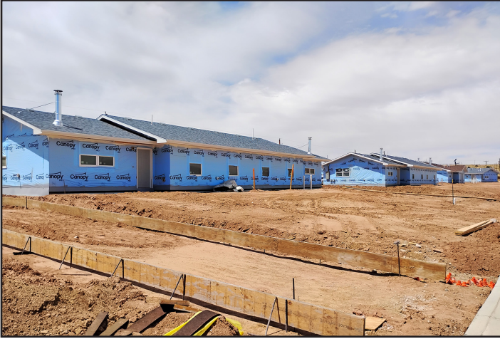
NM-15-047 in Crownpoint, a project for 50 public rental duplex units, is now moving to installation of curb, gutter, and driveways for the housing units.
