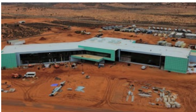
Area C – Glazing Curtain Wall (left wing). March 11, 2025.
