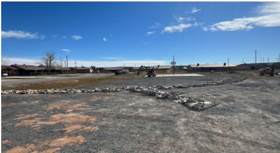
New Connex Storage Location
