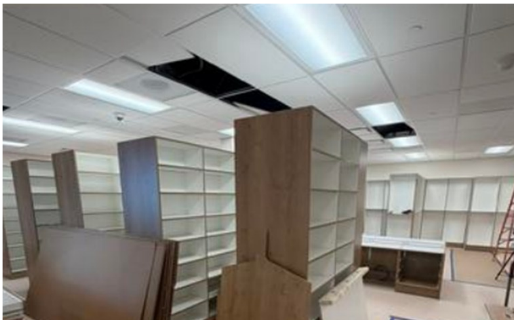
Pharmacy Equipment Installation
