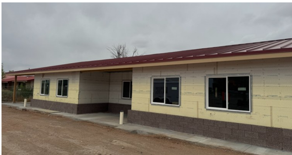
Staff Housing Unit Before Exterior EFIS Installation
